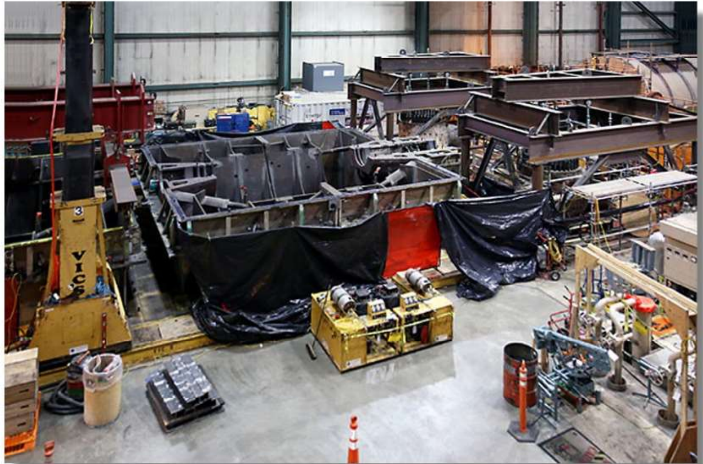
Shutdown of a plant due to a generator fire incident
